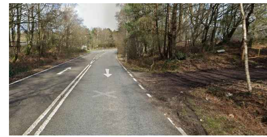
EXISTING ACCESS TRACK
