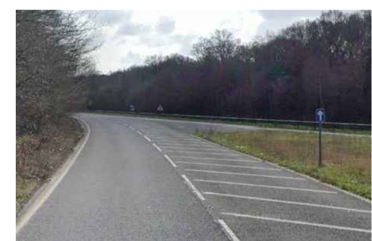
EXISTING ONE WAY SIGN
