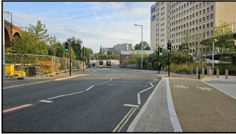
PHOTO 4 ASTLEY STREET LOOKING NORTH WEST TOWARDS HEATON LANE
